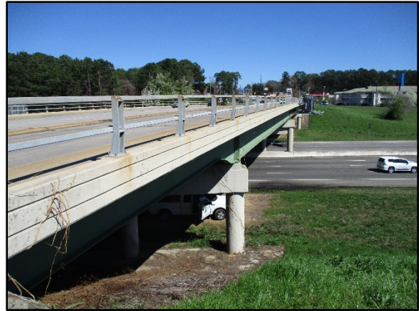
Photo 1 – S-40-36 (St. Andrews Rd.) Bridge over I-26 in Lexington County, SC.
